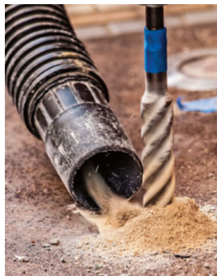
LEFT: Julie deciding where to place the sculpture RIGHT: Drilling Neolith, concrete, and rebar for a 9" bolt. Photos: Danny Fulgencio
